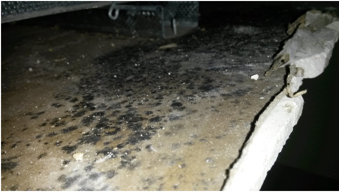
Water damage theatre roof
