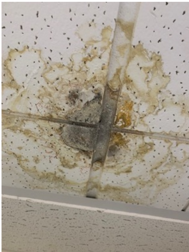
Ceiling in drug preparation area
