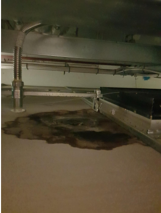
Water damage theatre roof
