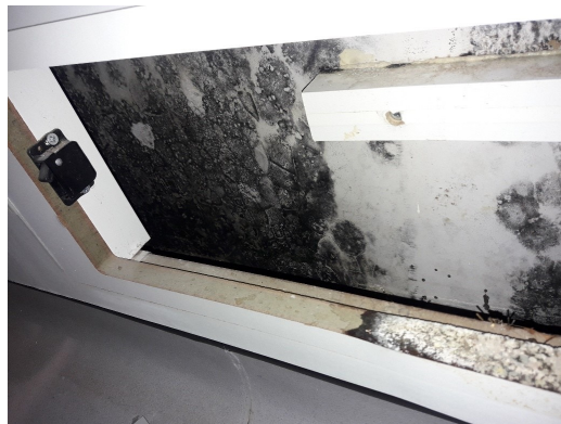
Ceiling void haemato-oncology unit
